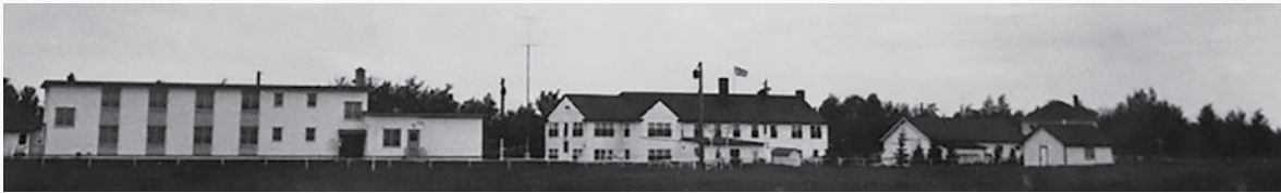
Fisher River Indian Hospital and nurses' residence. Detail from Library and Archives Canada/Department of Health fonds/e011052296.
